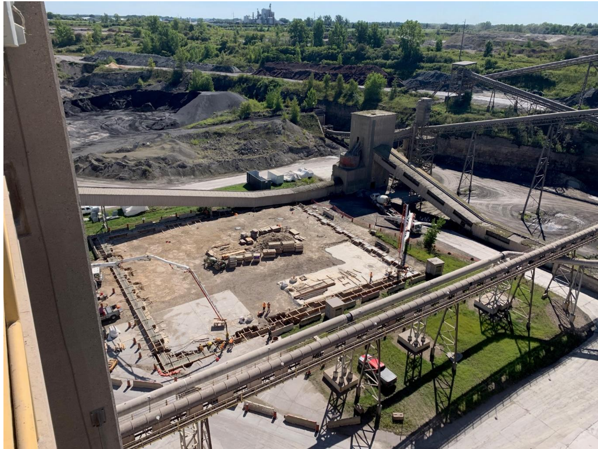
Alternative Low Carbon Fuels Building Excavation
