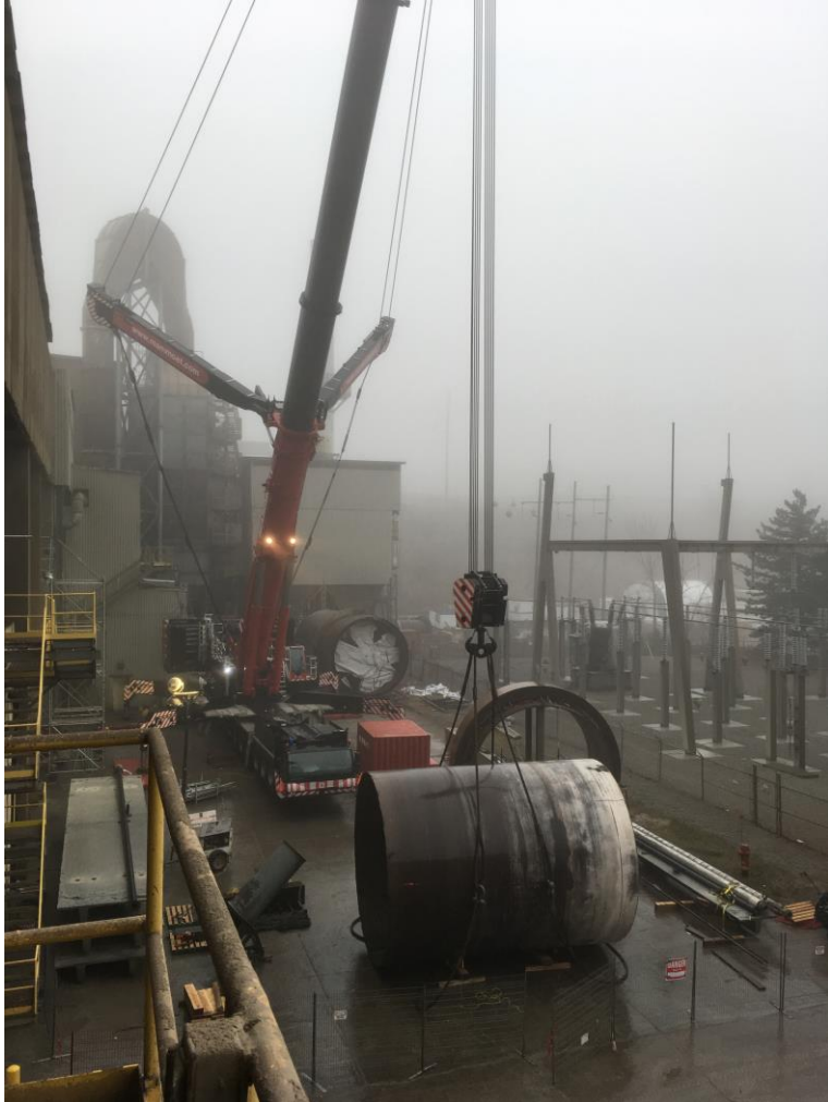
Kiln Shell Replacement 2017
