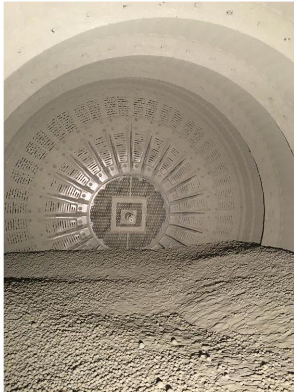
Finish Mill in Operation
